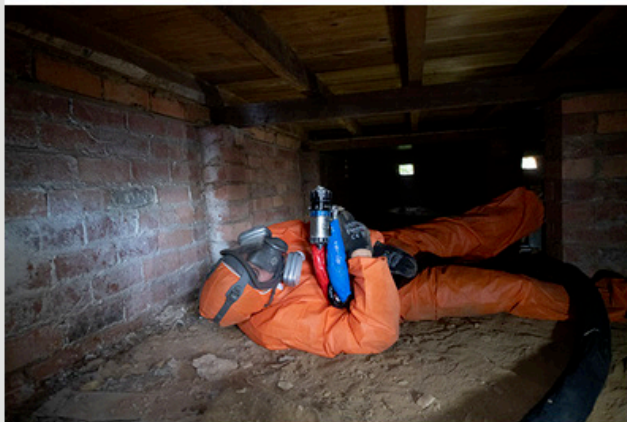
Applying closed cell spray polyurethane to the underside of the floorboards.
