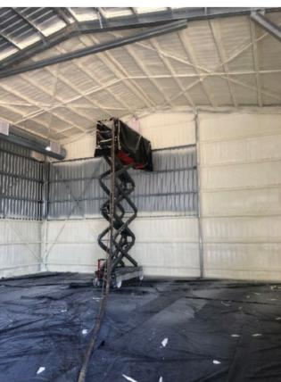
Agricultural sheds and buildings, garages, workshops or factories of any shape and size can also be sprayed with Polyurethane Spray Foam, creating a highly efficient thermal envelope.
